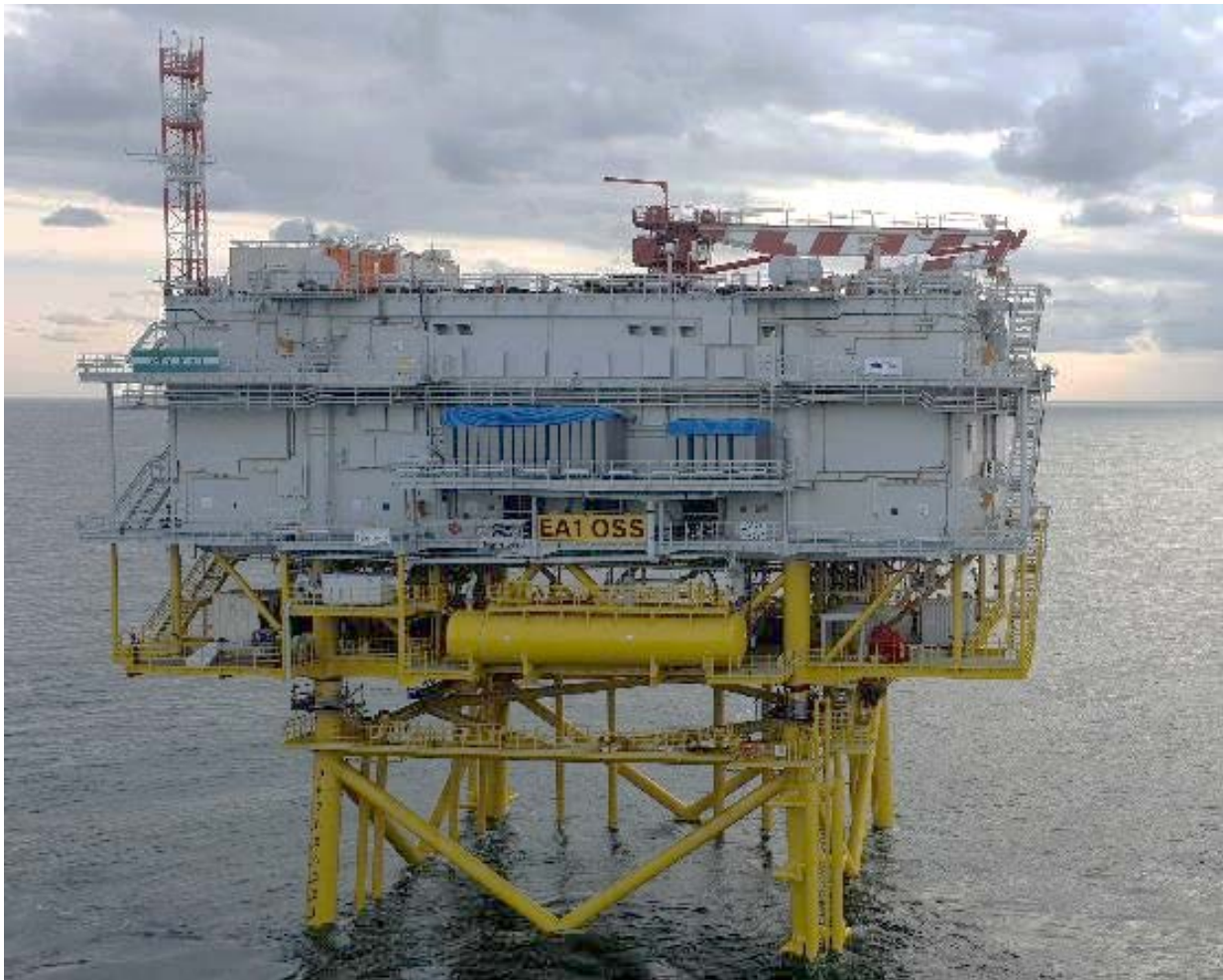
Plate 6.9 Typical Offshore Electrical Platform (AC collector station)
