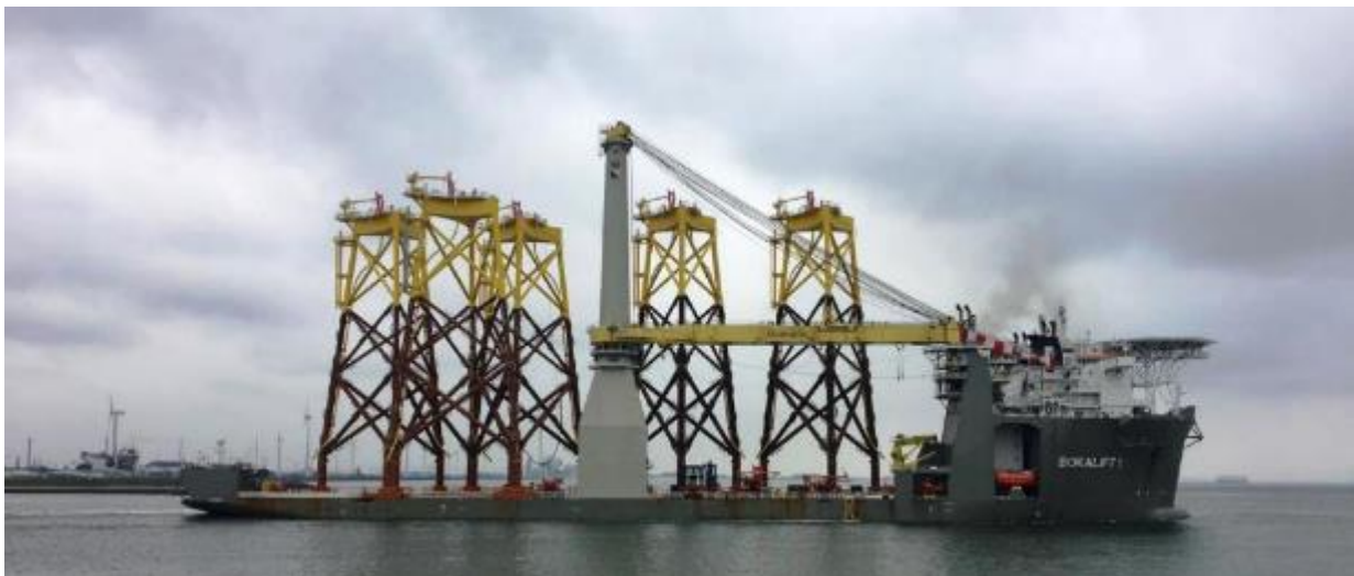
Plate 6.7 East Anglia ONE Three-Piled Jacket Foundations being Transported on a Heavy Lift Vessel
