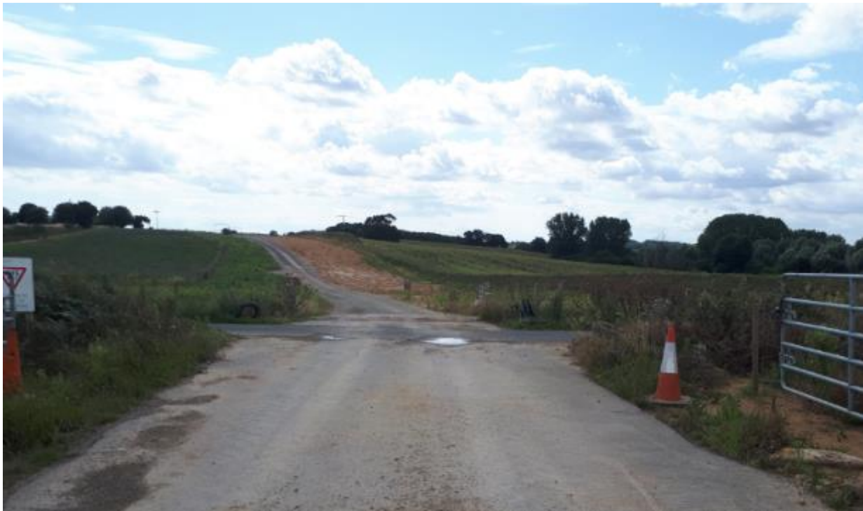
Plate 6.22 Example of an Onshore Cable Route Crossing of the Public Highway (image taken from East Anglia ONE project)
