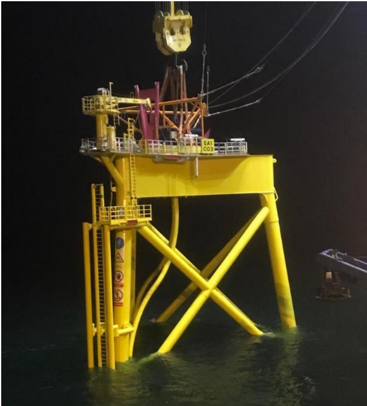
Plate 6.8 Three-Legged Jacket Foundation Part-Installed at the East Anglia ONE windfarm site
