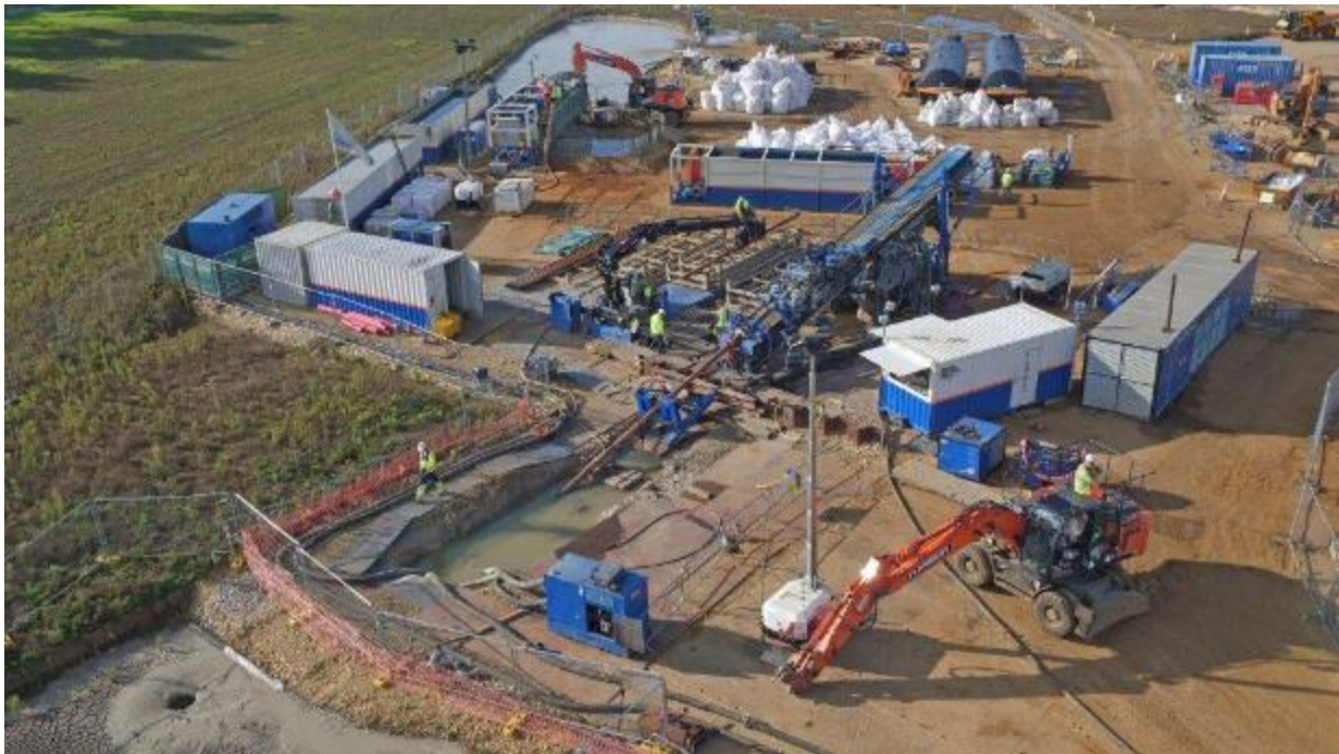
Plate 6.17 HDD landfall duct site (image taken from East Anglia ONE project)
